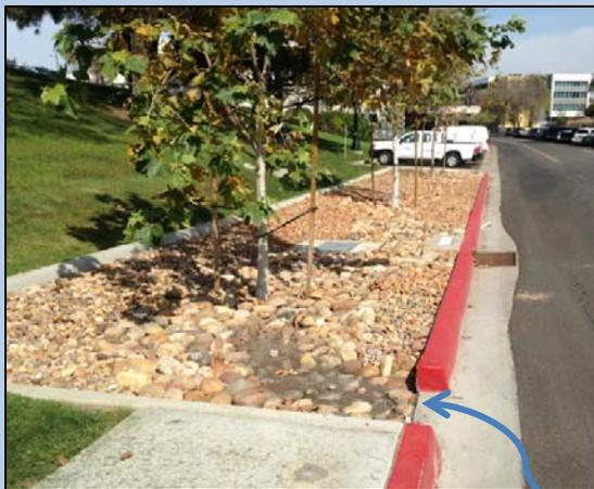
Storm water enters the basin from the street and is absorbed into the ground.
